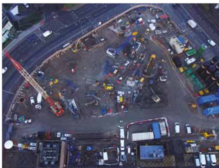
Aerial view of works on site
