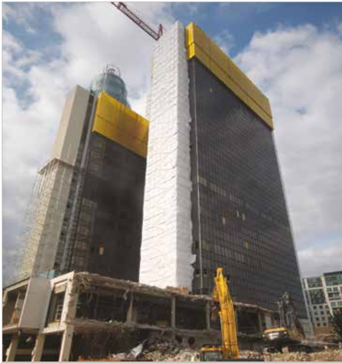
Use of Doka screens during demolition
